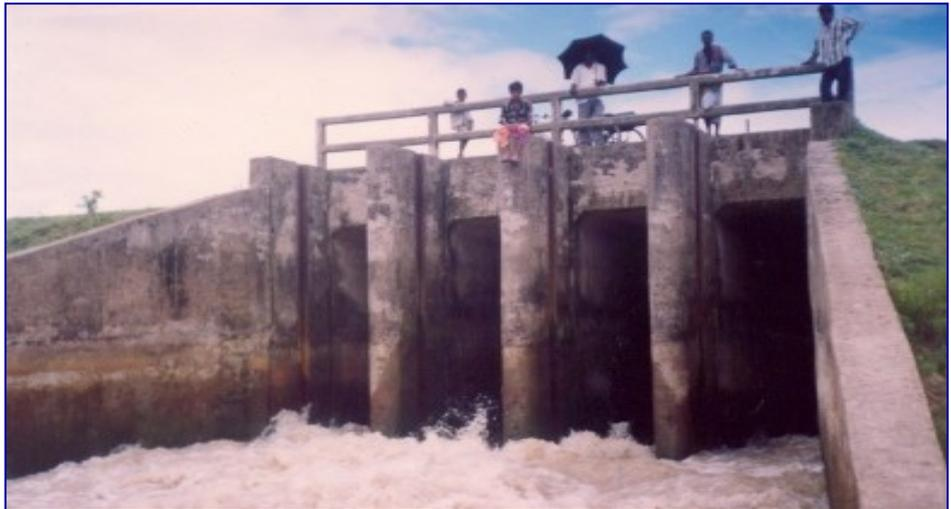
*A Sluice Gate in Bera Upazila, Pabna. Timely Operation of Sluice Gates is necessary for Fish Migration into Floodplain*
